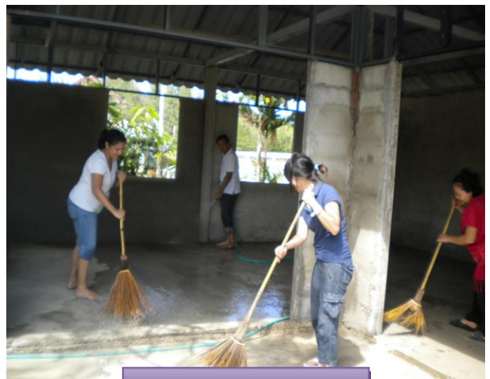
Getting ready for flooring
